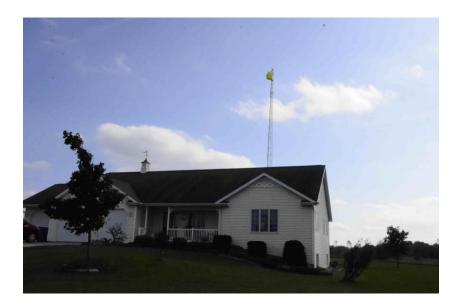
This documented the culmination of an entire summers efforts to locate a suitable tower, remove it from its previous location at Harry Harvey, N9AR's QTH, haul it out to Jim's, repaint it and perform other maintenance activities on it, hand dig a 4'x4'x6' hole for the antenna base, pour about 4cubic yards of concrete, and then reinstall the tower. A necessary, but not often documented aspect of our hobby.
