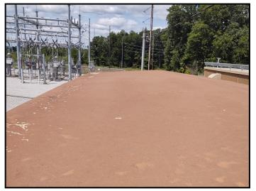
The crew applied a first coat of goop (Sealbest White Elastomeric Roof Coating) today as the initial step.
