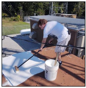
Sometime next week and second and final coat will be applied. Aside from sealing the roof, the new coating is white which should reduce the building air conditioning heat load during the summer.
