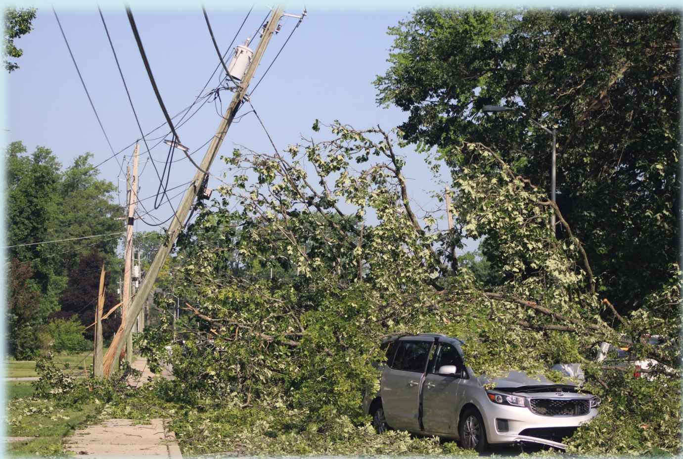
Tree, automobile and utility damage caused by the June 13, 2022, derecho in the Waynedale area of southwestern Fort Wayne, photographed June 14 by storm spotter Ashleigh Smoot. Photo used with permission.
